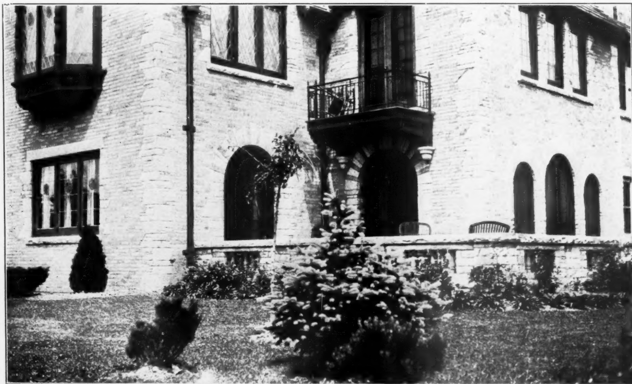
Palatial Home Made of Lannon Stone, Where Corners and Openings Have Been Emphasized by Special Trim
